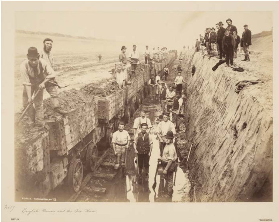
63* Manchester Ship Canal. A series of 17 photographs by Thomas Birtles (1832-1914), Warrington, c. 1887, albumen prints , showing scenes relating to the construction including some with navvies, images 25 x 35 cm, original card mounts with printed titles and credits to lower margins, numbered in pencil 1-17, original dark blue morocco gilt portfolio with remains of silk tie, a little split on joints, 45 x 57 cm overall (1) £300 - £500
