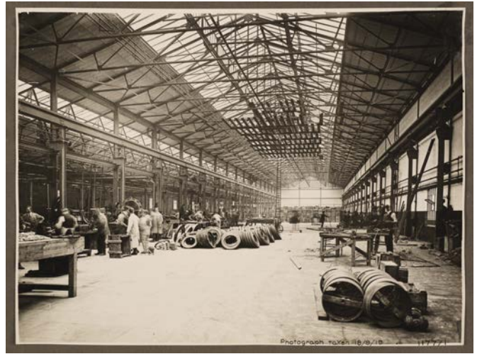
36* Dunlop Rubber . A collection of 90 photographs relating to the construction of a new factory at Fort Dunlop, Birmingham, England, mostly c. 1919–21, gelatin silver prints, some with negative numbers and dates printed in the lower margins, over 50 photographs pasted on to rectos and versos of album leaves, the remainder loose, mostly 21.5 x 29 cm but a few smaller including 2 panoramas, contemporary roan-backed buckram, rubbed and soiled, folio
